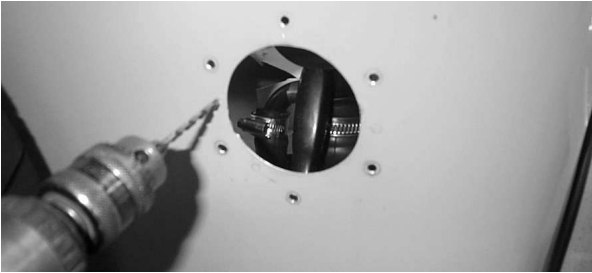
Fig 17 Carefully drill new holes
